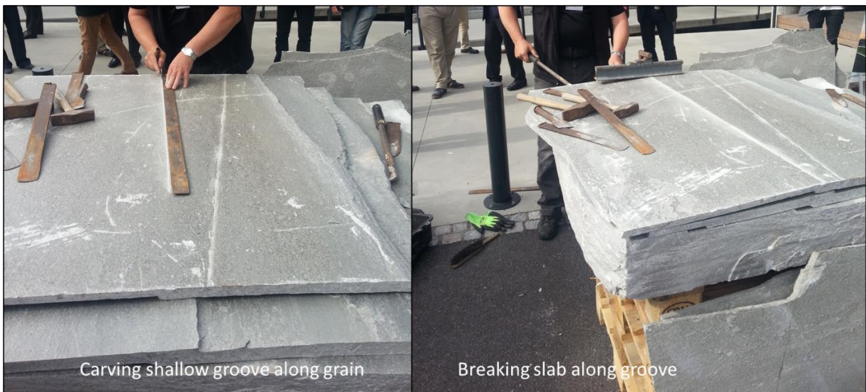
Figure 20. Breaking the slab in a rectangular shape.
