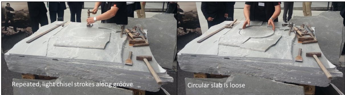
Figure 22. Repeated chiseling along the groove, loosening the circular slab.
