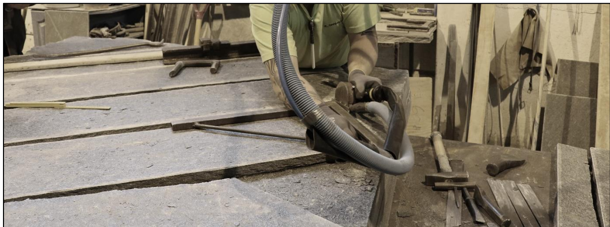
Figure 16. Pneumatic tools with diamond saw blade for making shallow grooves.
