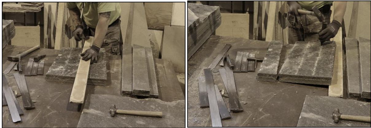
Figure 15. Breaking small slabs by chisel strokes along grooves.
