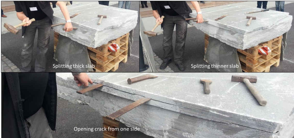
Figure 19. Making raw slab.
