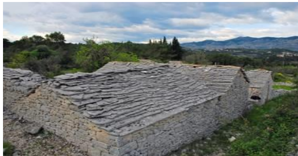
Traditional houses built of platy limestone at the Adriatic coast. Should they be abandoned and left to deteriorate? (photo delivered by Matevž Novak)
