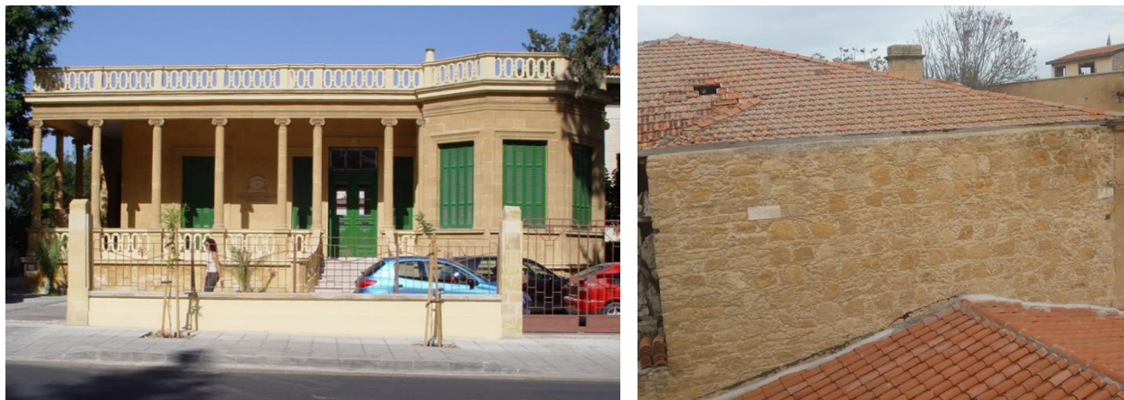
Fig. 16: On the left picture a listed house built exclusively with dimensional and ornamental stone. On the right the walls are built with irregular shape and size pieces of calcarenite.
