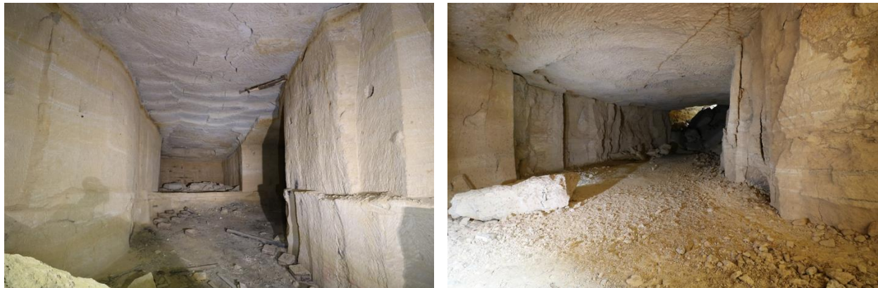
Fig. 19: Inside view of quarry landscape (cave) that shows cracks on the overlaying layers and on the walls.
