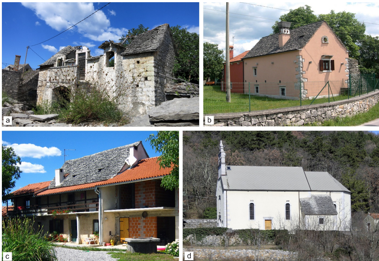
Figure 2. Bad practices in cultural heritage preservation and restoration. a Deterioration of stone-build house in Nakovana, Pelješac peninsula, Croatia. b Mimicking the vernacular architecture, Kras/Carso, Italy. c Mixing the roofing material, Kras/Carso, Italy. d Replacement of autochthonous limestone plates with industrial tiled covering, Saint Ulderico church in Sgonico, Italy. Reproduced from Novak (2015).
