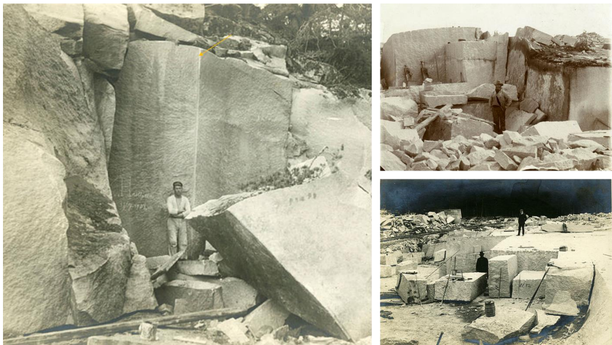
Figure 13. Left: single drill hole black powder blasting, releasing a large block of granite. Right: block reduction using horizontal and vertical wedging seems. All photos: NGU archive.
