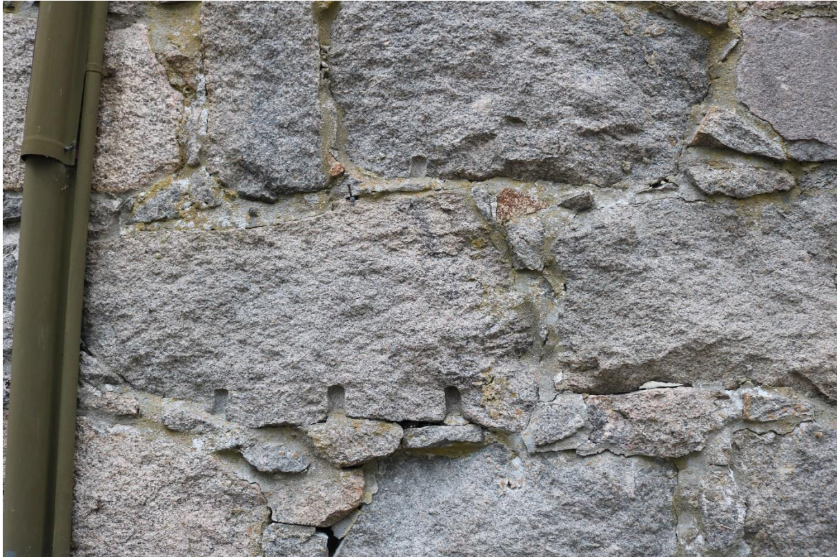
Figure 12. Fredrikstad Old Town. Granite blocks displaying marks from short and wide drill holes.
