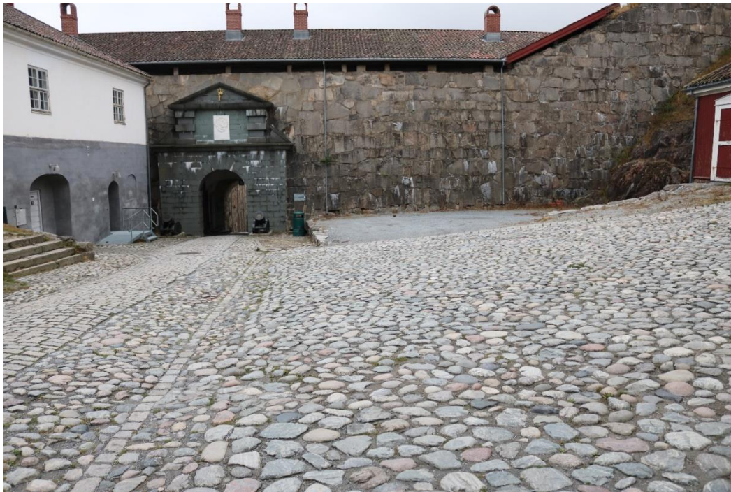
Figure 4. The Fredriksten Castle/fortress. Walls and paving stones predominantly made from the Iddefjord Granite.
