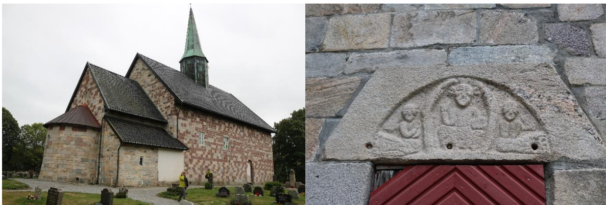
Figure 3. Rygge Church (1170 AD) is built predominantly of Iddefjord Granite and brownish syenite. Right: detail of relief carving in granite lintel.
